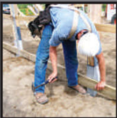
Attach Splash Board
